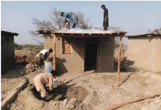
The construction of a new home made out of mud bricks in Pakistan. Photos: Fr Liam O'Callaghan SSC
